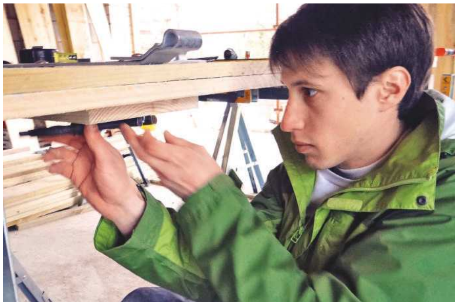
Aurélien bolts a hinge through three layers of wood with a lovely big old adjustable spanner Ed's had forever, and which often comes to his rescue. The hinge is cranked so that the door and the jamb with the pin on it sit flush
